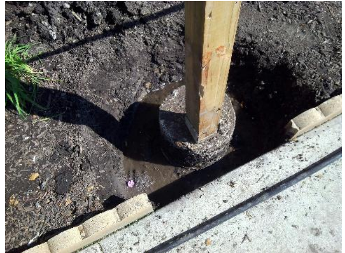
View of existing pier that was replaced during the repair project.
